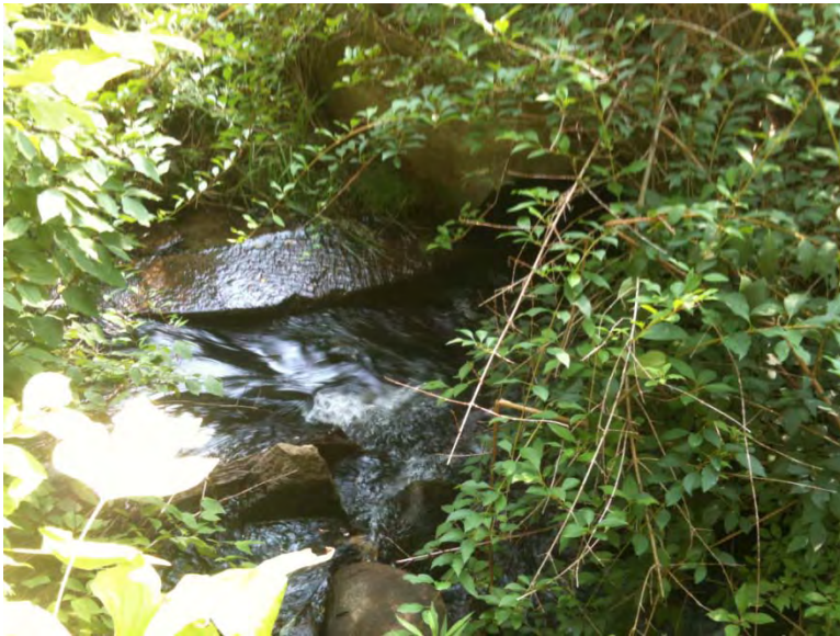
LOOKING UPSTREAM THROUGH PIPE
