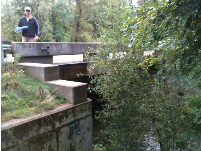
LOOKING AT CULVERT
