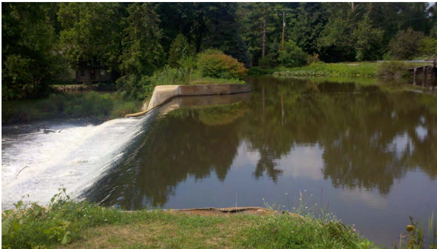
UPSTREAM OF KINGS MILL DAM
