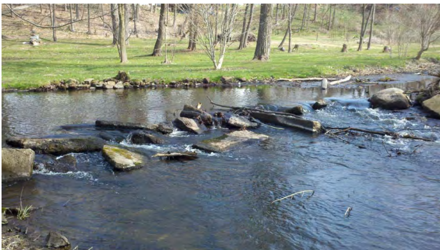
MCCOY DAM DIVERSION
