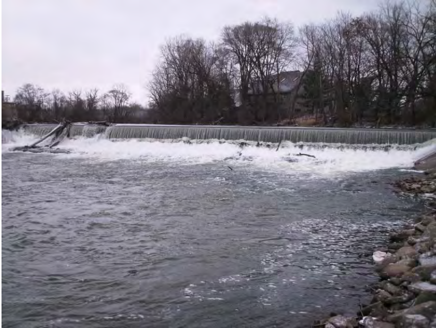
DOWNSTREAM ELKHART RIVER DAM
