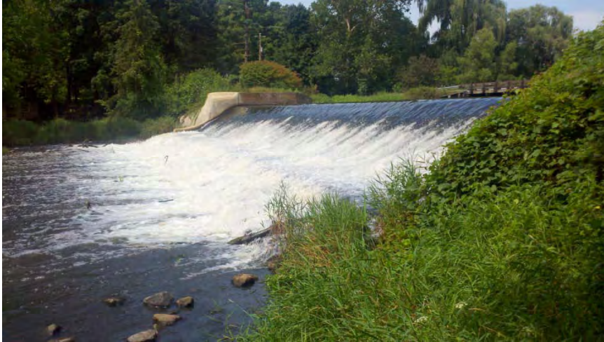
DOWNSTREAM OF KINGS MILL DAM
