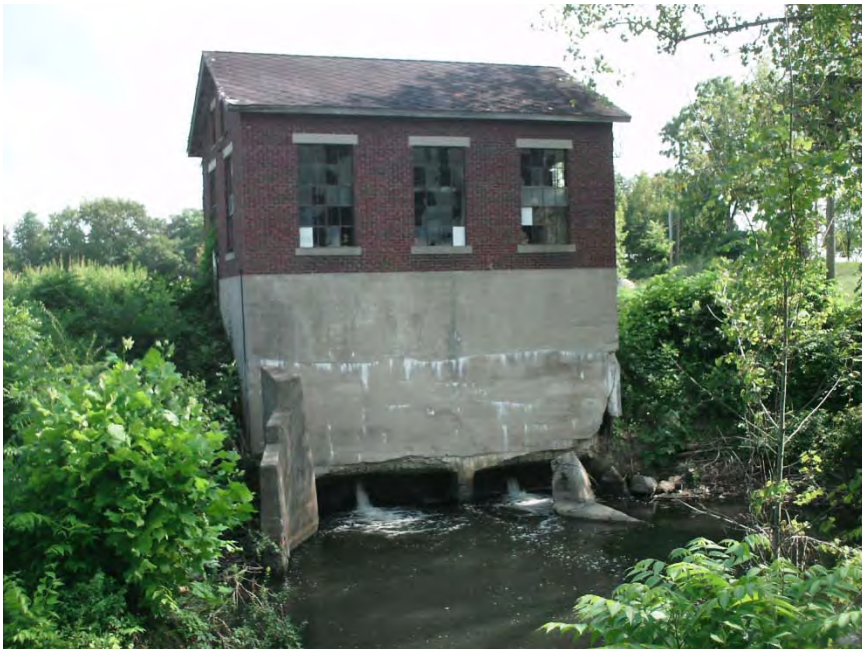
STAR MILLING HYDRO PLANT
