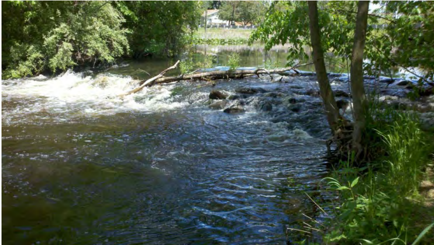
LEONIDUS ROLLER MILL DAM, SOUTH BYPASS
