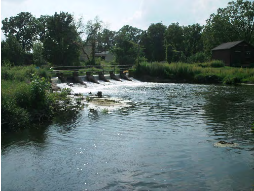
DOWNSTREAM OF STAR MILLING DAM
