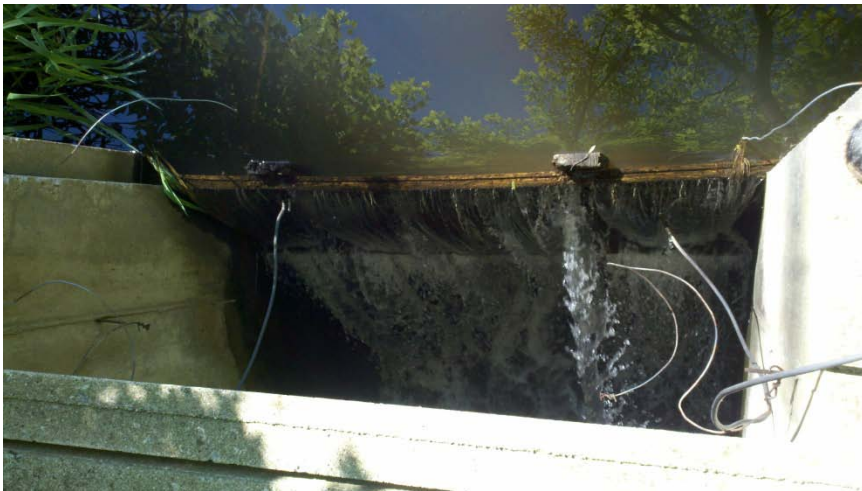
MEYER DAM FROM TOP
