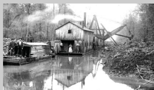
Dredging Machine on the Kankakee River (www.gokankakeeriver.org)
